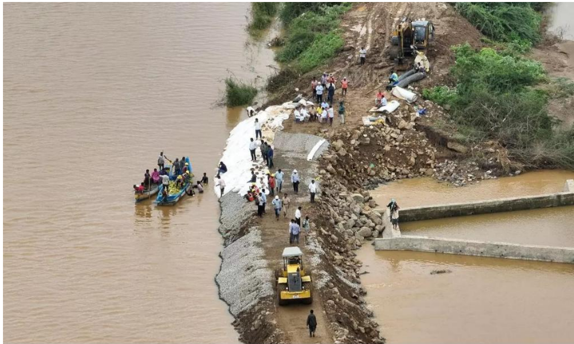
Fig 2. Plugging the breach of Budameru, a rivulet. Source: (Nagaraju, 2024)
